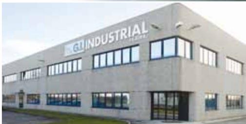
Rivignano Teor – ITALY. Production Plant.
