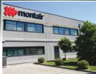
Piove di Sacco – ITALY. Close Control Business Unit and Production Plant.
